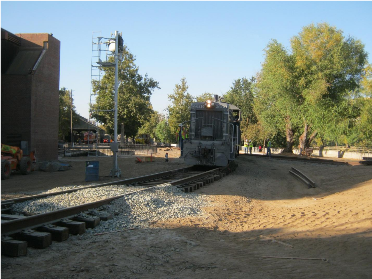
First train over the new track!
